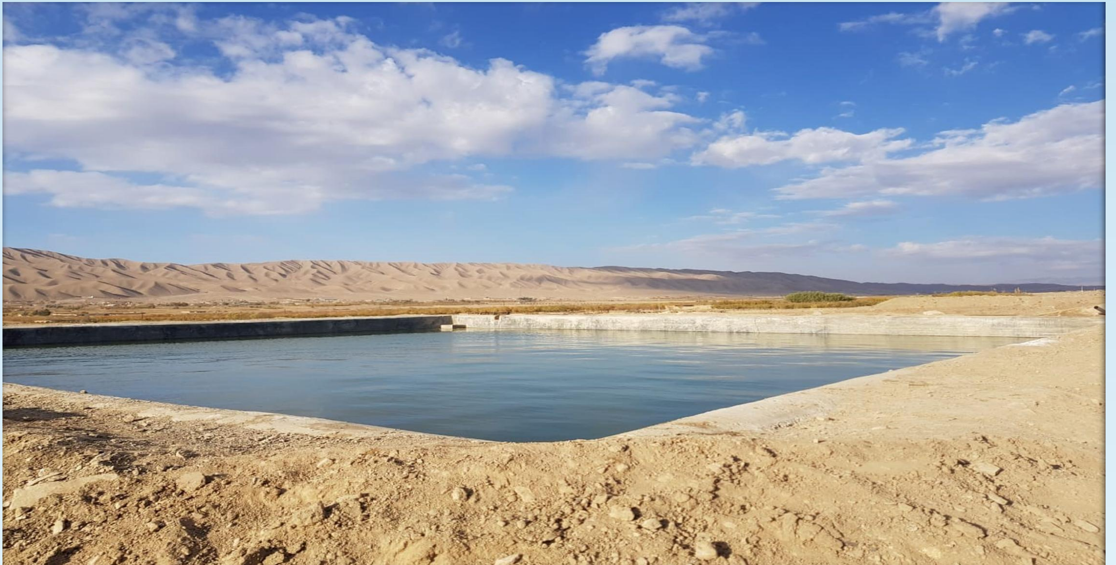
Killa Abdullah-Women-led water reservoir constructed in UC Purana Chaman
